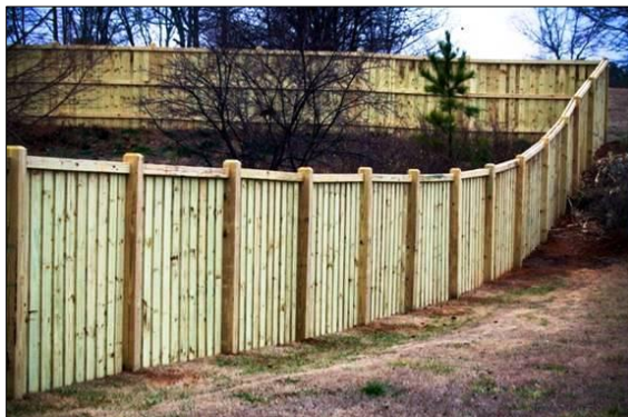
Figure 5-17: Fence with Finished Side Out
